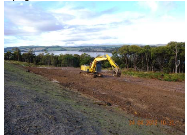
Plate 2 – Scarification treatment of disturbed areas in progress
