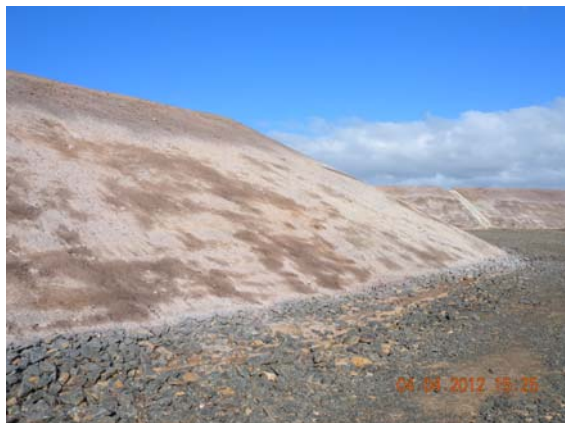
Plate 1& 3 - Hydro-seeded and BFM treated batter
